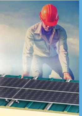
Thanks to its special clamp system, Solar Capped Panel is easily mounted on the surface of Assan Sandwich Panel without drilling any screw holes. As it is installed without drilling on the roof, it offers excellent waterproofing performance and high corrosion resistance as well as extending the economic life of the buildings by maintaining the structural integrity of the roofs. In addition, it offers cost efficiency in steel construction with its design allowing for low slope
