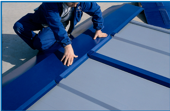
5- Assembly of ridge
