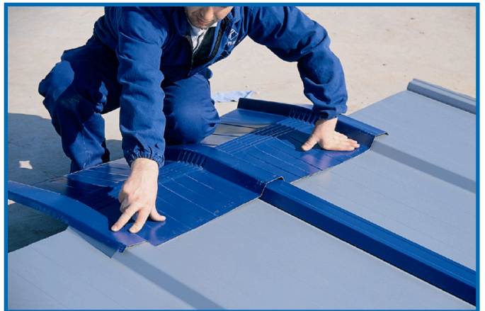
6- Assembly of ridge with radius
