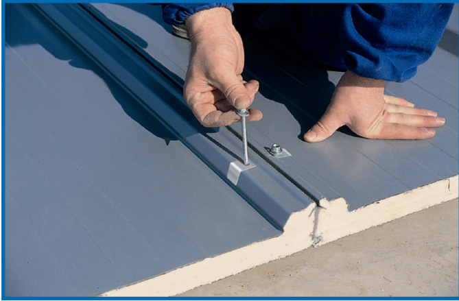
1- Assembly of Screws
