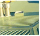
The polyurethane-filled sandwich panels have the adequate sound absorption characteristic in the normal industrial buildings according to the requirement of the building; however, they are not sufficient for the regions or offices that are very sensitive to sound and therefore additional solutions such as vibration absorbers may be required.
