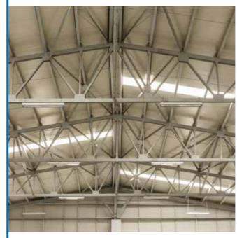
curves. Standing seam roof sheets are supported directly off the roof purlins via the support clips/halters.
